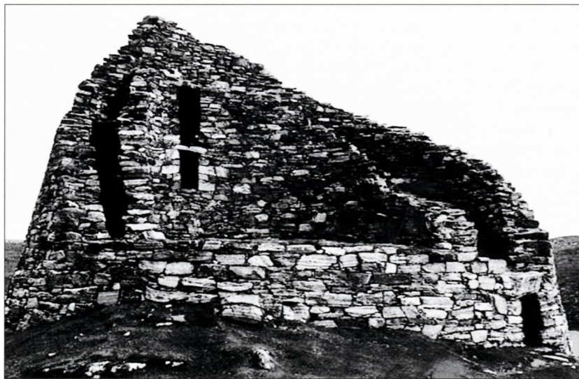
Dun Carloway (Dun Charlabhaigh) is another small but well-preserved Late Iron Age broch, whose remains perch spectacularly above Loch Roag on Lewis. The broch was damaged during a 16th-century Highland feud when it was used as a hideout, but the double-skinned nature of its wall construction is all the more clearly shown by the ruinous condition. (Historic Scotland)
