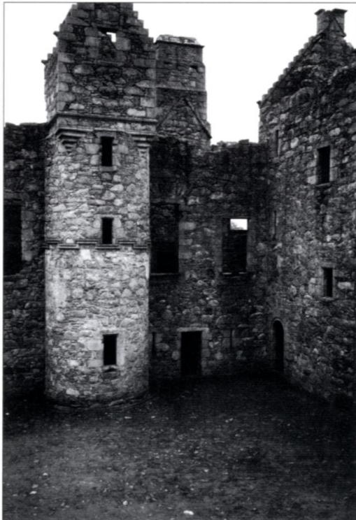
Tolquhon Castle: the main domestic range. As is often the case the prominent tower is not a defensive feature, but simply houses a stairway.
