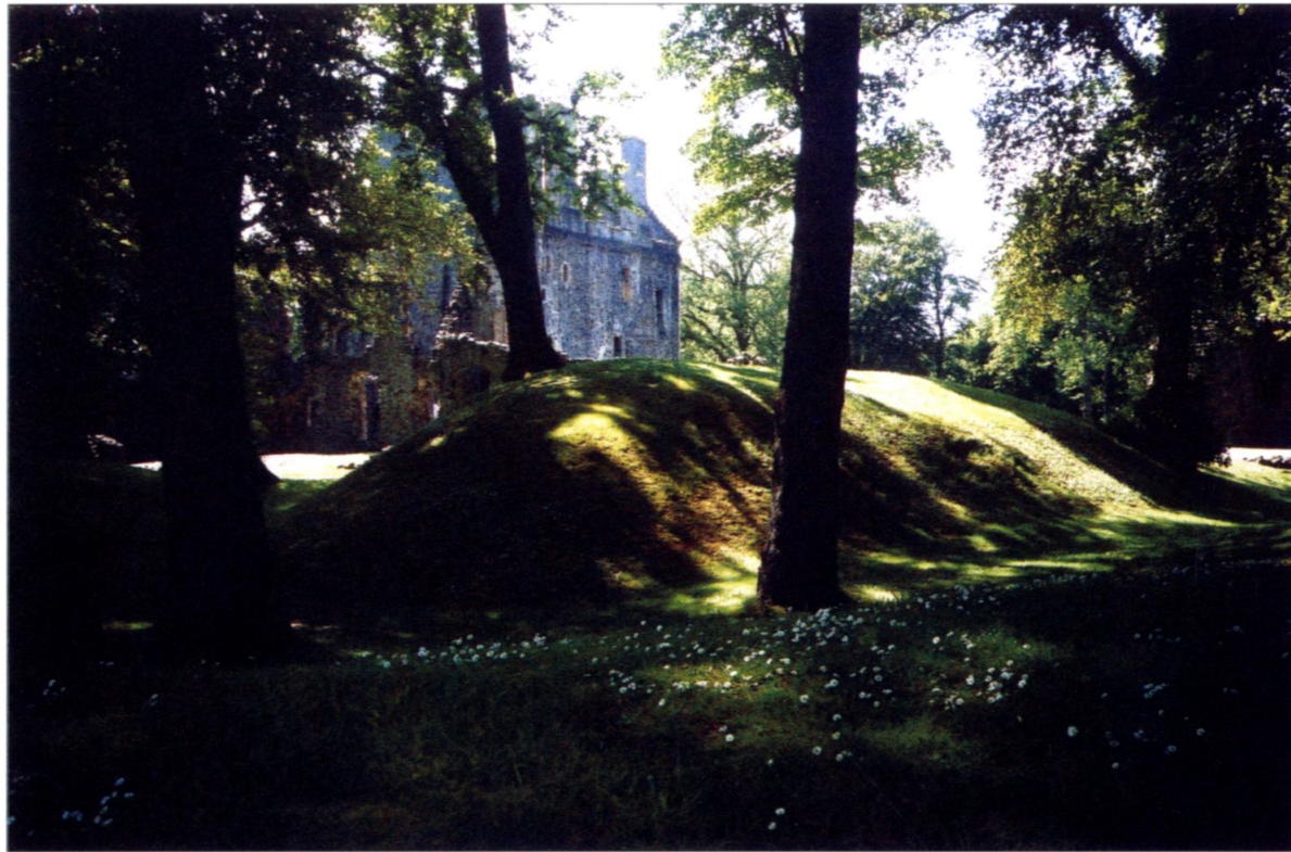
ABOVE As a rule Scottish castles were not designed to withstand artillery fire; this earthwork ravelin constructed at Huntly Castle during the Civil War period is thus extremely rare.
