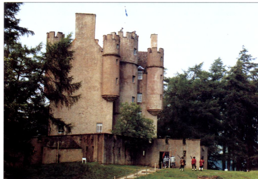
Braemar Castle is perhaps the quintessential L-plan tower house. Although the present loop-holed outer wall, like the near identical one at Corgarff, was actually constructed by the British Army after 1746, the tower house will almost certainly have been surrounded by an earlier barmekin wall of similar dimensions.
