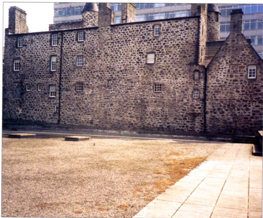
TOP RIGHT Provost Skene's House, Aberdeen. The original part of the building, dating from 1545, was a fairly modest L-plan tower house, seen at the left of the photograph. Subsequent building work in 1626 and 1669 not only extended it to the right and raised it by another floor, but also added another, taller L-plan tower on the end. The arched gateway is a much later addition transplanted from a quite different property.
