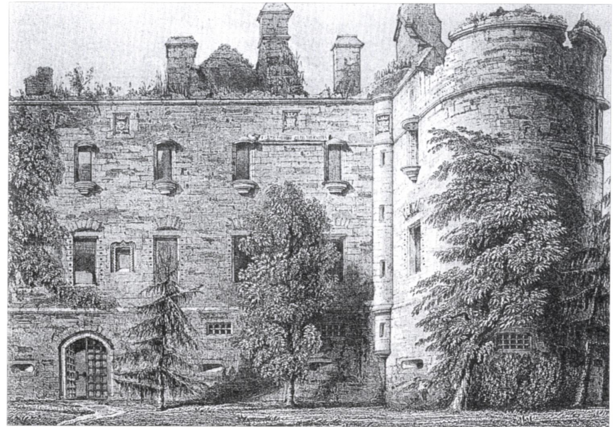
The L2 'hall' tower at Balvenie Castle engraved by R.W. Billings for the Baronial and Ecclesiastical Antiquities of Scotland (1845–52). Note the large gunloops running around the bottom of the wall.
