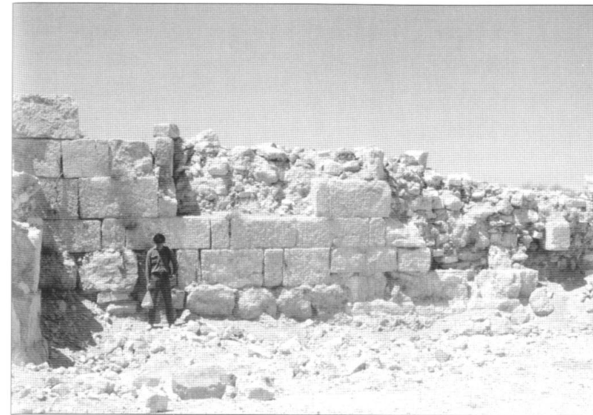
At Udruh (Jordan), the massive walls, c.3m thick, consist of a rubble core faced with limestone blocks, and still stand to a height of 6m in some places. (© M. C. Bishop)
