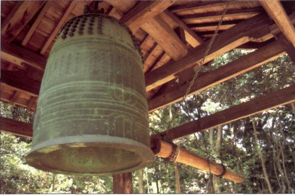
The bell at Negorodera. As in all Japanese examples, the bell hangs inside the bell tower, and is rung by using a heavy wooden external clapper, which is swung by a rope.
