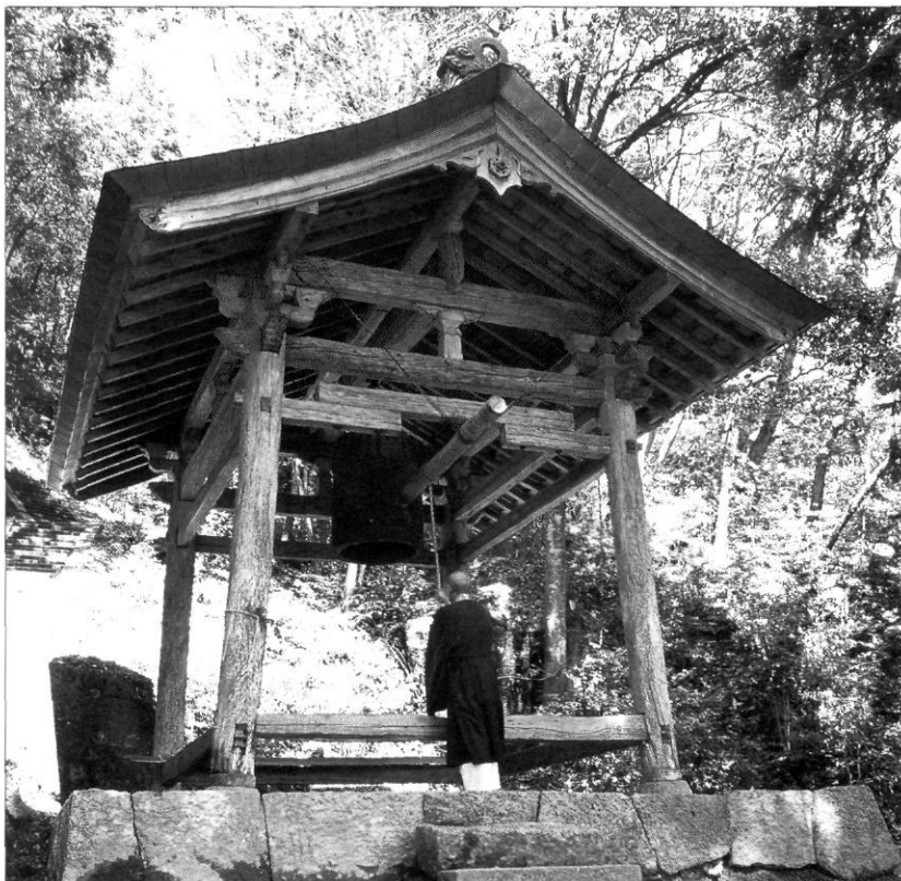
The bell tower of Sokusoji, a Tendai mountain temple in Mie Prefecture. This is a typical Japanese bell tower based on the design of a simple wooden frame beneath a protective roof.
