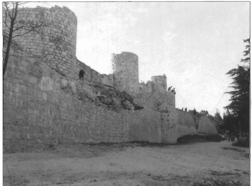
The strong walls of the eastern side of the castle of Burgos are pictured here. No attacks were made against this section of the walls.
