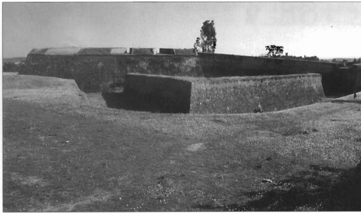
Fort San Cristobal, Badajoz, as seen from the covered way. The glacis rolls away behind the camera, effectively shielding all that is visible in this photo. It is a most effective glacis.
