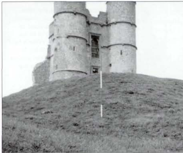
Earthen bastions constructed by the Royalist garrison in 1643 in front of the gatehouse at Donnington Castle near Newbury, Berkshire. It is quite probable that such earthworks were surmounted with wooden palisades and other obstacles.
