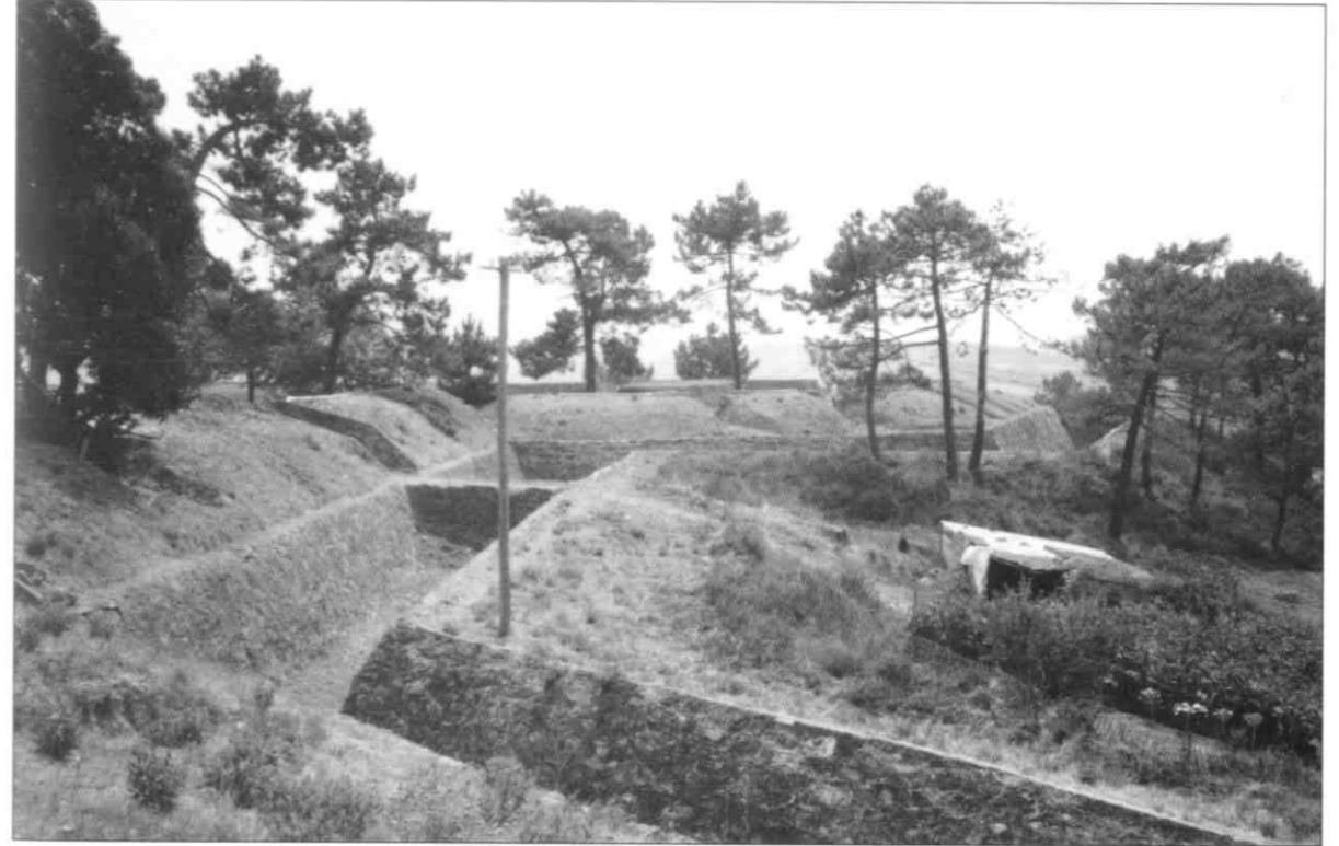
Fort San Vicente, Torres Vedras. A fine view of the ditch, glacis and the ramparts of the fort. It was constructed in such a way as to cover the approaches, and is a fine example of the way in which engineers turned away from the elaborate star-shaped forts of the previous century. The ditches and interior walls have been somewhat artificially preserved with concrete. It serves as a focal point for commemoration of the Lines of Torres Vedras.
