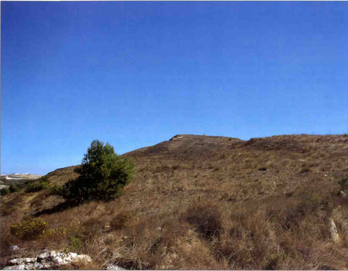
Another view of fort number 40, clearly showing the way in which it covered the surrounding area. The steep approach would have made it difficult for the French to attack, whilst any attempt to outflank it would have been parried by the two forts nearby, 41 and 42.
