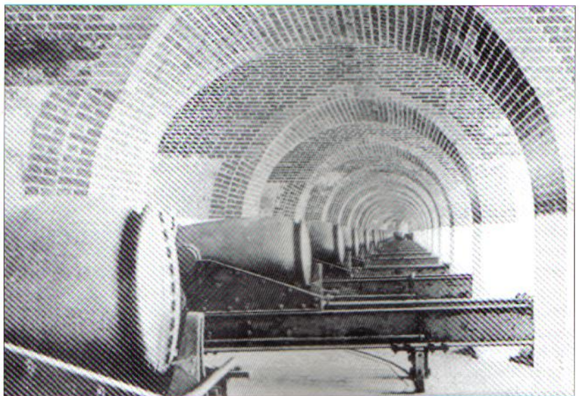
Smoothbore columbiad pieces mounted on iron casemate carriages in the water battery of Fort Monroe, Virginia, photographed shortly after the Civil War. Note the unusual color scheme of the fort, where the lower casemate walls have been painted white. (Estate of Wright Langley)
