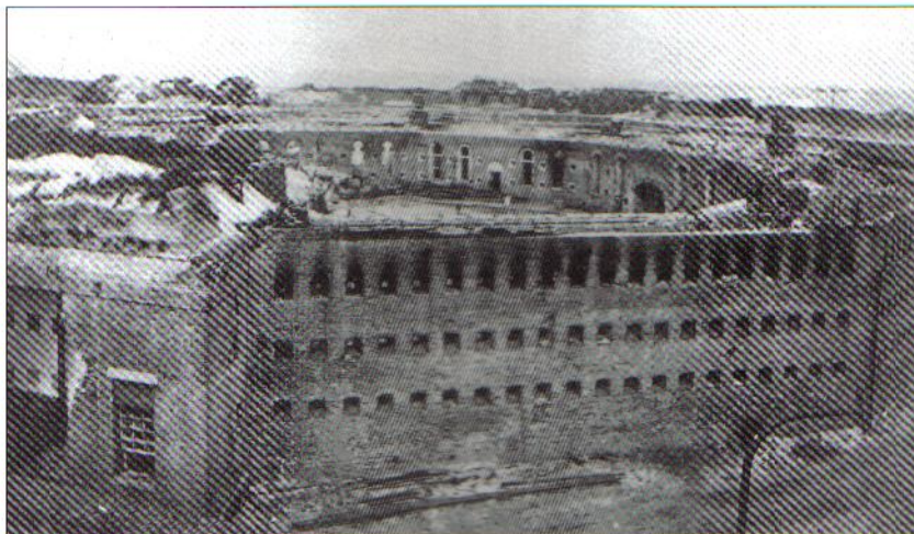
Fort Morgan, Mobile Bay, Alabama, photographed from the nearby lighthouse after her surrender to Union forces in August 1864. The damage inflicted on the fort by the Union fleet was concentrated on the upper works, and the southwestern seaward scarp. (Salamander Archives)
