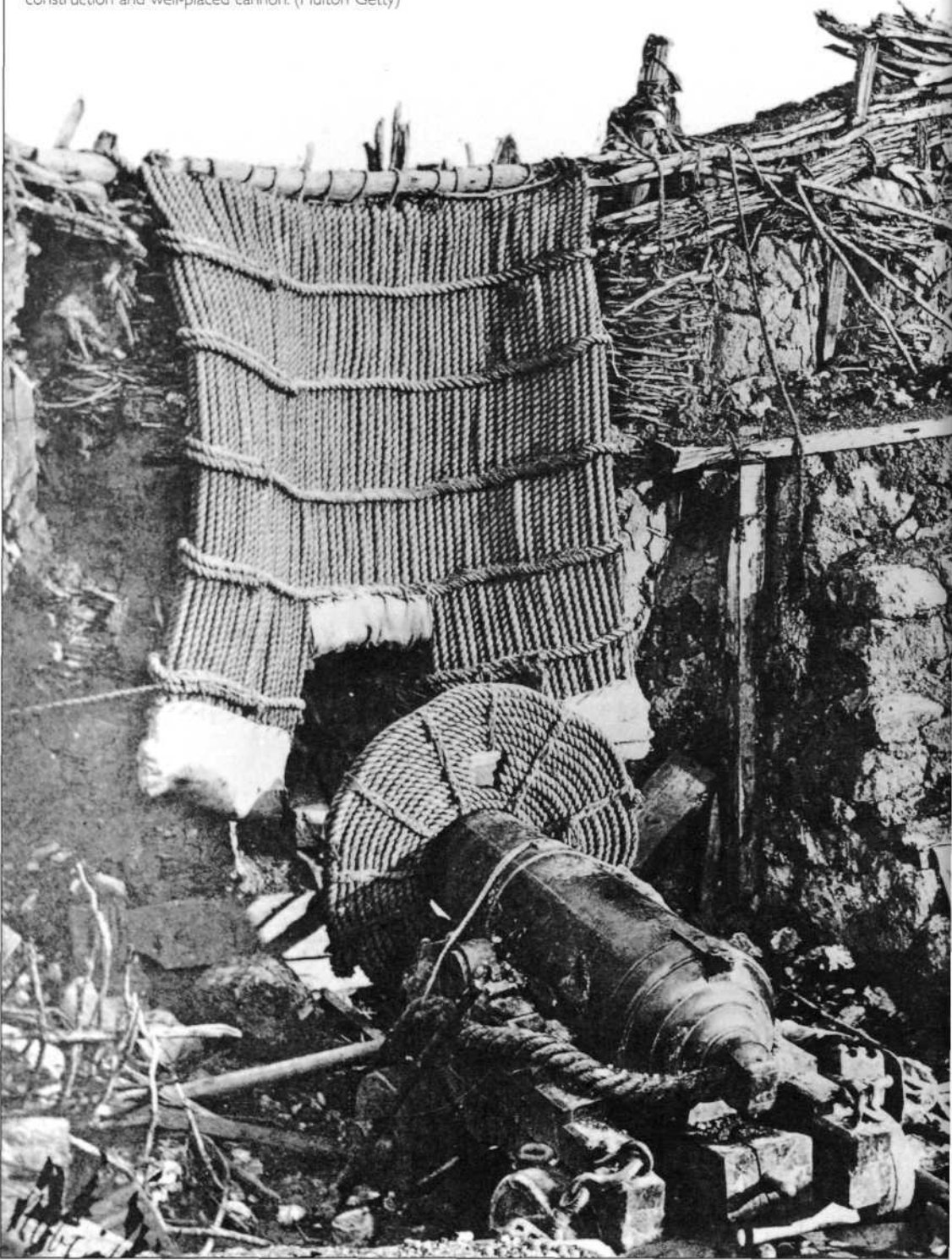
The Great Redan. Interior of the earthwork, photographed after the Russian withdrawal, showing its formidable construction and well-placed cannon. (Hulton Getty)
