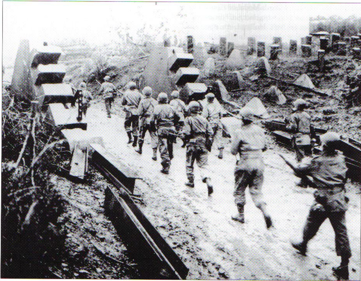
American infantry advance through a section of the Siegfried Line. The line was littered with a variety of obstacles to stop tank attacks, such as the "Dragon's teeth" to the right of the road and the pair of ramps each side of the road designed to force tanks to expose their lightly armored undersides. (NARA)
