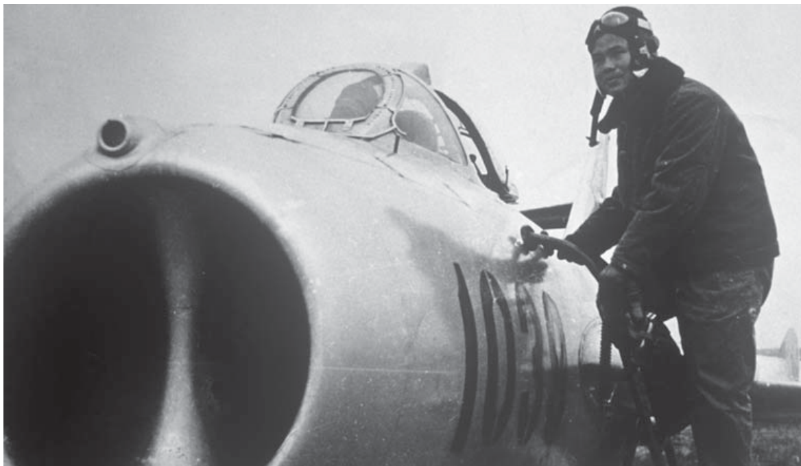
A pilot boards his MiG-17 “Fresco-A” (almost certainly a Chinese-built Shenyang J-5) using a short ladder. The circular port above the main intake is the fighter’s gun camera, a similar device being seen in this location on the MiG-15 and MiG-19. (via Dr István Toperczer)
