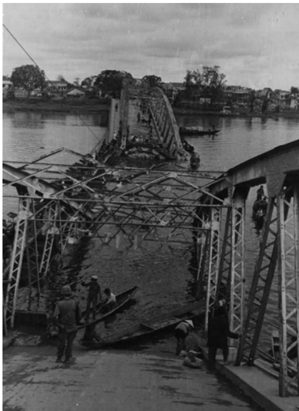
February 28, 1968: Looking south along the multispans bowstring girder Nguyễn Hoàng Bridge, part of Highway 1. Marines attempted to cross to the Citadel's Thượng Tứ Gate, when heavy NVA fire forced them back to the southern bank. On February 7, enemy sappers triggered explosives that dropped a span into the Perfume River. Note the pontoon foot bridge at left. (Cummins (Marine Corps))
