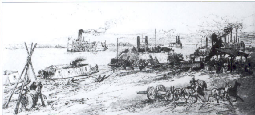
"United States Mississippi Gunboats being built at Carondelet, near St Louis, Missouri." Engraving published in Harper's Weekly , October 5, 1861. Although somewhat inaccurate, it purports to show the construction of the wooden frames of four of the City class vessels. (USNHC)
