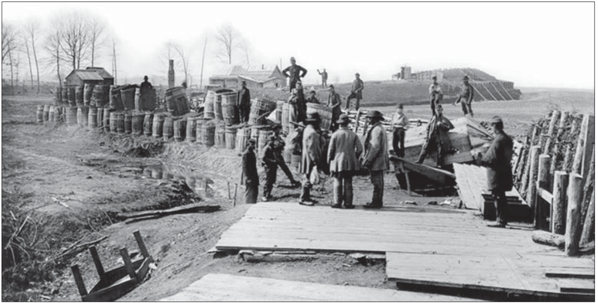
Captured Confederate fortifications at Manassas, Virginia in 1862. The remains of a gabion revetment can be seen in the middle ground. A vertical post revetment protects the battery in the background. (Library of Congress B817-7936)
