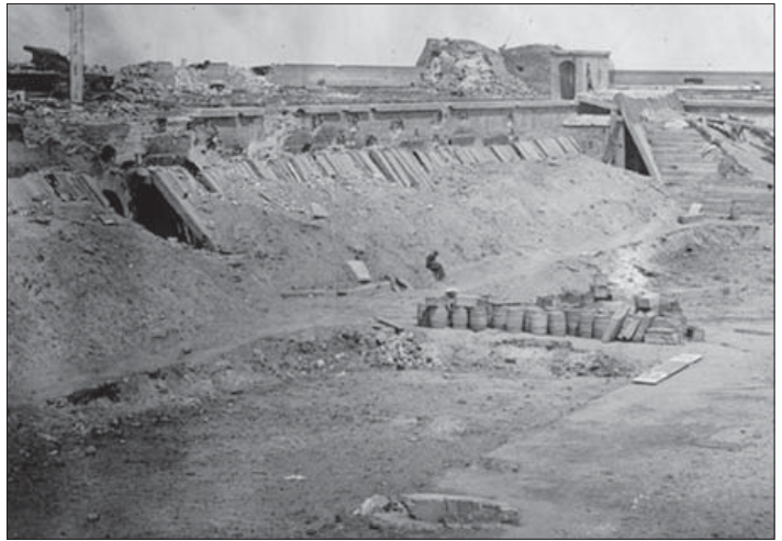
These casemates were found covered by heavy timber blindage after the capture of Fort Pulaski by Federal forces in April 1862. (Library of Congress B8171-0194)
