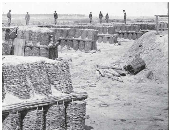
These impressive gabionade traverses along the interior slope of the parapet forming the right face of the right redan of Fort Sedgwick (nicknamed "Fort Hell") were photographed on April 3, 1865. Fascines are placed between the two layers of gabion. Note the empty gabion lying by the bomb-proof shelter. (Library of Congress B8171-7693)
