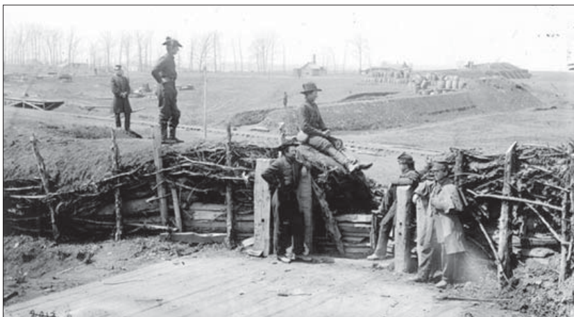
Photographed after capture in 1862, these Confederate field fortifications at Manassas, Virginia consisted of a hurdle revetment behind an earthen parapet with an embrasure. Note the artillery platform in the foreground. (Library of Congress B817-7171)
