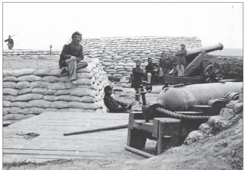
Sandbags provided the traverses for this Confederate redoubt captured at Yorktown in April 1862. A 32-pounder seacoast gun stands nearest the camera, while a 24-pounder siege piece on a wooden barbette carriage is seen nearby. (Library of Congress B811-2366A)
