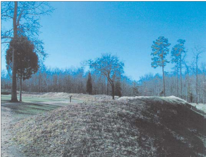
Originally forming part of the exterior line of Confederate defenses surrounding Richmond, Virginia, the substantial earthwork remains of Fort Harrison are today part of the Richmond National Battlefield Park. (Courtesy of Richmond National Battlefield Park)
