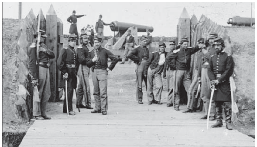
Soldiers standing at the gate of Fort Slemmer, one of the enclosed forts constructed to the north of Washington, DC. Note the wide wooden ramp that gave access across a deep ditch. The siege gun in the rear stands on a wooden barbette carriage. (Library of Congress B811-2318)
