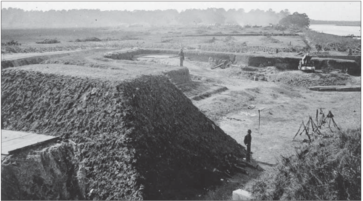
A view of the interior of Fort McAllister, Savannah, taken after its capture by Federal forces on December 13, 1864. The large parapets traverse standing in the foreground was designed to limit the area affected by explosions that might occur within gun positions during heavy and prolonged bombardment. The entrance work at bottom left also indicates that it probably served as a bomb-proof shelter or powder magazine. (Library of Congress B81 I-4004)
