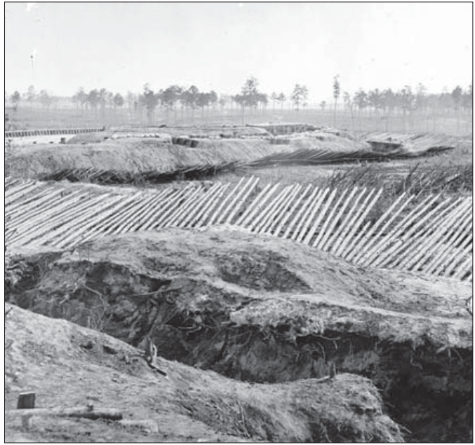
Taken from Fort Sedgwick outside the Petersburg lines on April 3, 1865, this photograph shows a fraise and deep ditch in front of the breastworks. (Library of Congress B811-3209A)
