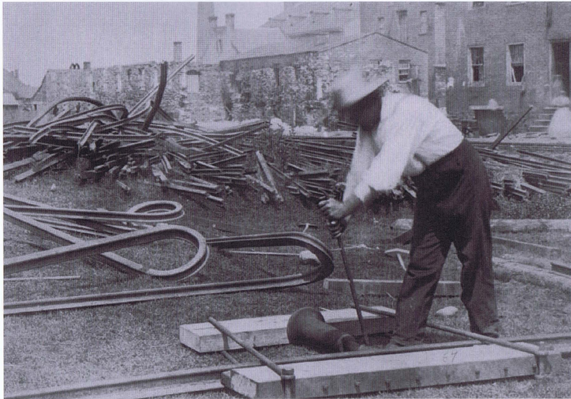
This man is re-straightening bent rails with a jackscrew. There was no universal specification, and "T-rail" track varied in weight from about 35lb to 68lb per yard. (LC)
