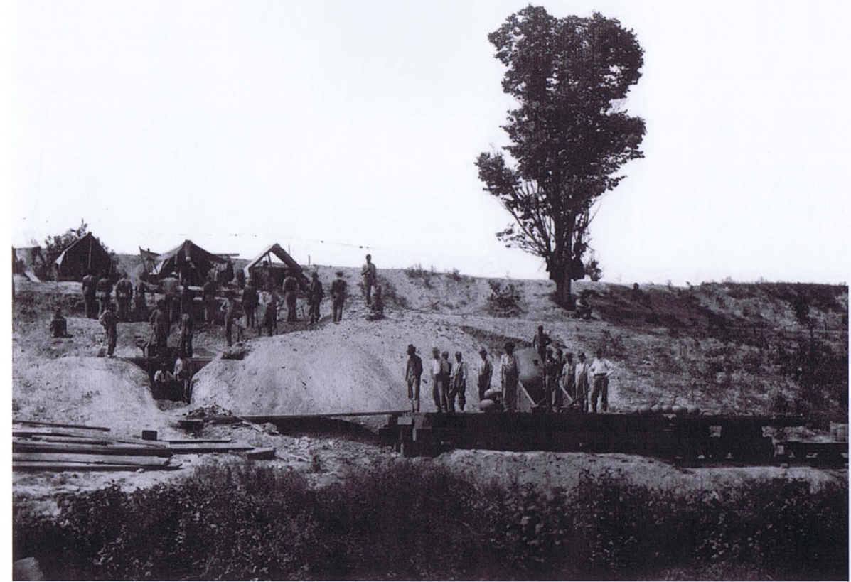
A blurred but rare image of the Dictator in position. Just visible at far right is a pole car carrying three powder kegs; ahead of it the mortar's taller four-axle transport car butts up against the mortar platform. Left of the end of the foot plank, two men stand in the doorway of a munitions bunker cut into the hill; this bunker can still be seen today. (LC)
