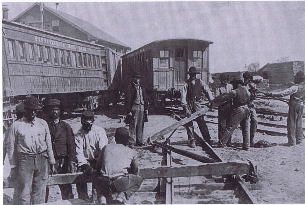
Members of the USMRR Construction Corps demonstrating how to twist rails using hooks and levers. Notice that the men working under the supervisor in civilian dress are black laborers, not white soldiers detailed for the job, so this photograph was taken after BrigGen Haupt had established his permanent workforce. During the war, Northerners typically referred to all black people, free or slave, as "contrabands." Note also the passenger cars in the background. (LC)
