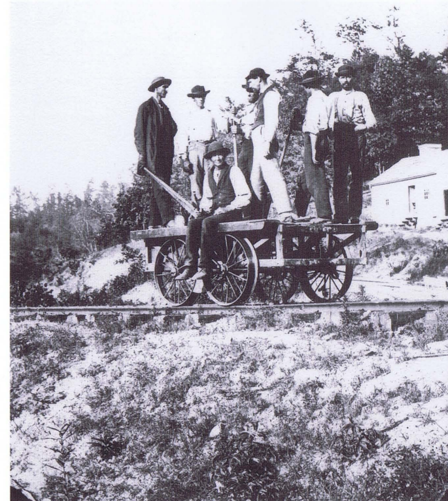
Several workmen riding down the tracks on a lightweight handcar. At center, note the men grasping the protruding levers (visible as pale uprights) that work the gearing connected to the axles. The man in the dark coat is probably grasping a brake handle. (Courtesy B & O Railroad Museum)
