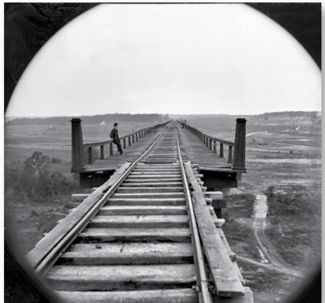
The tracks of the Southside Railroad stretch about 2,400ft across the High Bridge. In this O'Sullivan photograph, the photographer poses at left while his assistant operates the camera. (Library of Congress LC-DIG-cwpb-01299)
