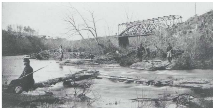
The railroad bridge near Union Mills remained intact, allowing Federal rolling stock to continue along this section of the Orange & Alexandria. LC
