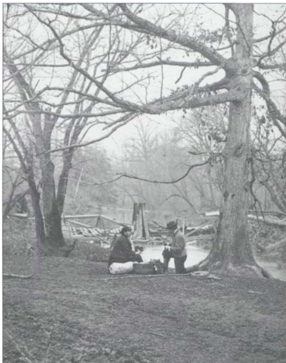
These ruins of the railroad bridge at Blackburn's Ford are typical of the damage inflicted during the efforts made by both sides to disrupt the enemy's lines of communications. LC
