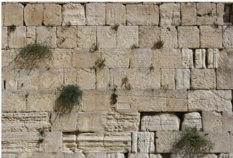
The retaining wall on its western flank is all that remains above ground of Herod's Temple Mount. The massive stone blocks are mute testament to its grandeur – and the challenge it presented to the Roman besiegers. (Author's Collection)
