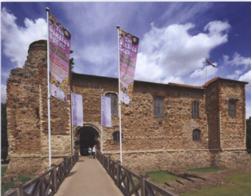
Colchester Castle stands foursquare upon the remains of the lofty podium of the massive temple of Claudius. Completed by around 1100, the Norman builders also took tiles and stone from this and the ruins of other Roman buildings in the town. Though now only two storeys high, the keep was once even bigger than its London counterpart, the Tower. (George Gastin)
