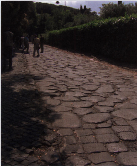
The Via Appia, which connected Rome with Campania, Lucania and Apulia, was the first and most spectacular of the consular roads. As far as Terracina, a distance of 62 Roman miles, it ran in an almost entirely straight line, even through the Alban Hills, where the gradients are steep. Here we see the well-paved stretch just beyond the Tomb of Cecilia Metella, Parco Regionale dell'Appia Antica. (Fields-Carré Collection)
