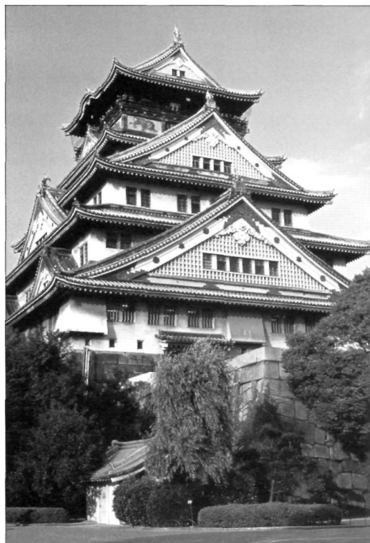
The keep of Osaka Castle, rebuilt according to the dimensions of the original keep that saw the siege of Osaka.
