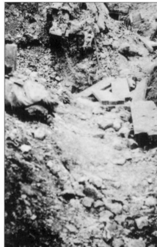
A German trench in La Boisselle captured by the British on 1 July. Of note are the pre-cut timber boards used to support mine galleries and dugout entrances, which were a feature of the German defensive system. (Courtesy of the Director, National Army Museum, London)
