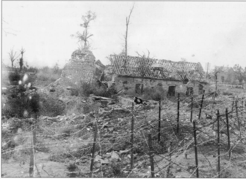
A German barbed-wire defence as captured near Mametz. This photograph demonstrates the sophistication of barbed wire in which a double row of stakes has been linked to form a dense entanglement. On the attacker's side an apron pegged to the ground prevents the upright wire from being easily cut. This is a formidable obstacle to infantry. (IWM Q4181)
