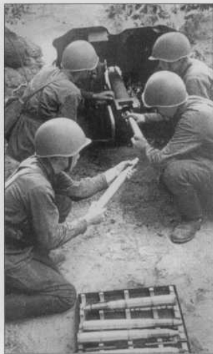
In 1941, each Soviet rifle regiment had an anti-tank battery with six 45mm M1937 anti-tank guns. Here, the crew is loading UO-243 HE-FRAG rounds but the primary ammunition was the UB-242/243 series APHE-T round. (Nik Cornish)
