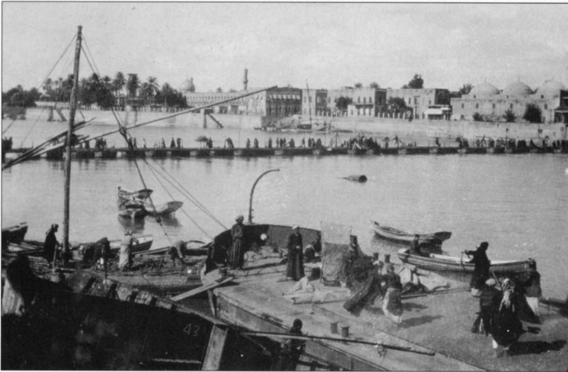
The Khota Bridge at Baghdad. (F. Webb via RAF Habbaniya Association)
