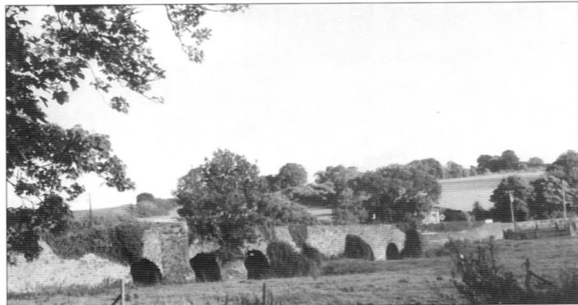
The Magdalene Bridge at Duleek. After both Jacobite wings had begun to withdraw, the army's survival came down to who could reach the bridge first. Wide enough to take six men marching abreast, the bridge formed a bottleneck that could have resulted in the destruction of the Jacobite army had the Williamites been able to mount a serious pursuit. (Author's photograph)
