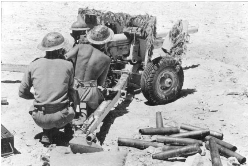
British 6-pdr anti-tank gun in action. The arrival of the 6-pdr in North Africa in mid-1942 gave the British a powerful weapon with which to finally counter German tanks. Its 2.84kg shell could penetrate 50mm of armour at 1,500 metres. (IWM E15559)
