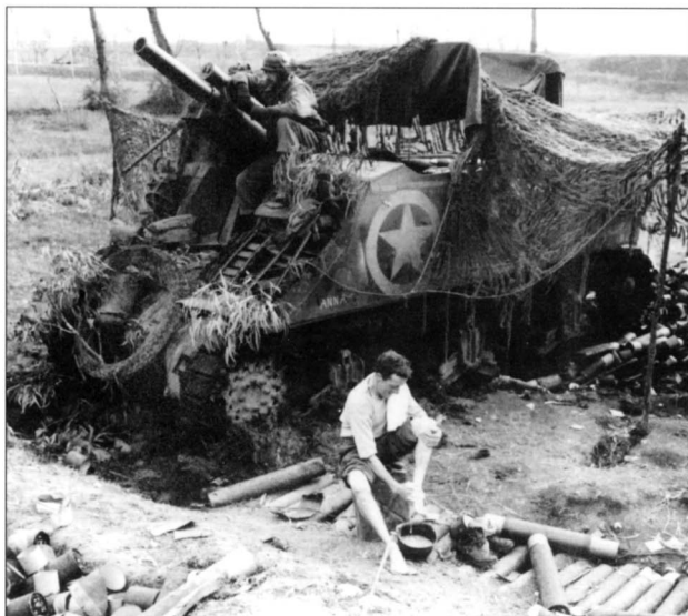
An M7 105mm howitzer motor carriage named Anna of Battery A, 69th Armored Field Artillery Battalion, 1st Armored Division in firing position near Nettuno on 2 February 1944. There are numerous empty ammunition packing tubes near the howitzer from heavy firing. (NARA)
