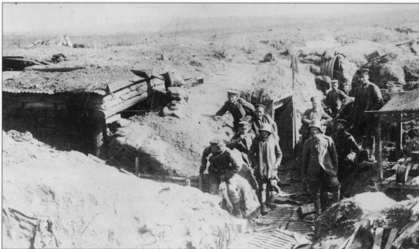
A German reserve Stellung on the Somme. It might appear to be in poor repair but the bunker and dugout are looking solid enough. Note all the field telephone cable. (IWM, Q23931)
