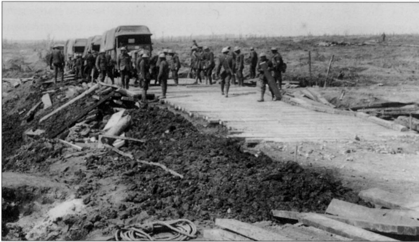
Plank road being constructed on Vimy Ridge. In preparation for the attack, Canadian Corps Labour Companies built 10km of plank road. (IWM, CO 1261)
