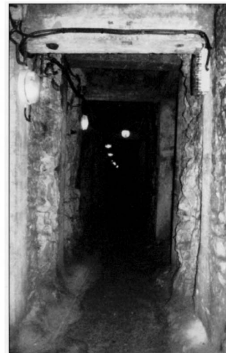
The Grange Subway as it is today. Omit the plastic lights; replace concrete with timber and it is completely unchanged. The glass insulators just visible above the left-hand light fixtures were for telegraph and field telephone communication cable. Chalk could conduct the traffic to enemy listening devices. (Author's collection)
