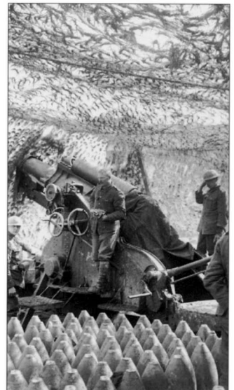
A 9.2in. howitzer on the Arras front, 1 April 1917. The recoil of this weapon was sufficient to topple it over so designers fitted a removable 'earth box' to the front end. A classic piece of civilian design intervention in the procurement process, this box took 12 hours of spadework to fill and had to be emptied again by hand when the gun moved. (IWM, Q6460)
