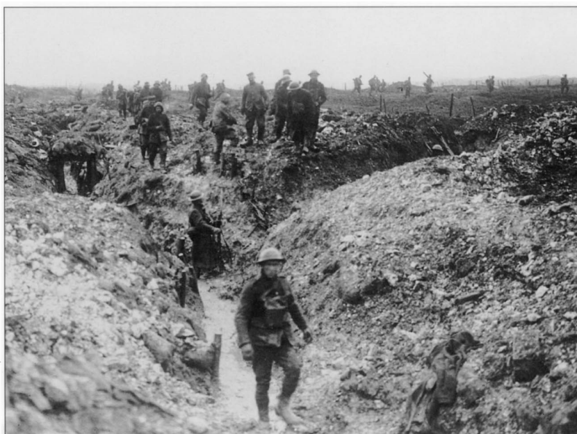
Canadians guarding German dugout entrances. The overhead protection is designed to prevent the entrances from becoming blocked by shellfire. In many cases, men were entombed and across Vimy Ridge, the Germans paid a high price for placing so many men into single dugouts. (IWM, CO 1154)
