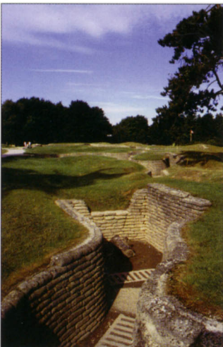
The German Minenwerfer emplacement in the preserved outpost line of Vimy memorial park. The outposts themselves are forward of this point and the Canadian flag marks the approximate position of the Grange Subway exit. (Author's collection)
