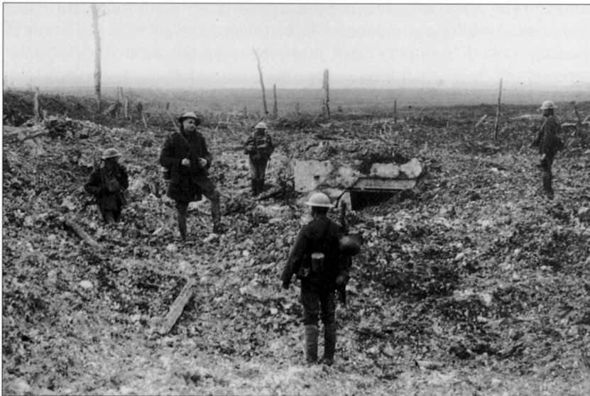
The Arras-Lille road atop Vimy Ridge. We will have to take the photographer's word for it. The chalk fragments, buried concrete strongpoint and total eradication of the road is further evidence of the effect achieved by an entire army's scaling of heavy artillery in such a limited area. (IWM, CO 1145)
