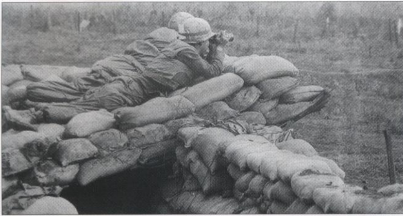
A pair of Marines lay atop their perimeter bunker searching for the faint telltale puff of smoke of a mortar firing. This was extremely difficult among the vegetation, dust, and fog. The three-sandbag-thick roof is laid atop recovered M18 airfield matting. Draped over the sandbags are firing wires leading to M18A1 Claymore antipersonnel mines in the barrier wire.
