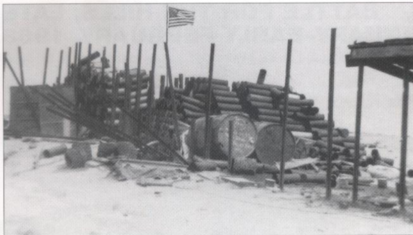
With the American flag flying defiantly above it, what appears to be a heap of discarded ammunition tubes and 55gal drums is actually the combat operations center for I/3/26 Marines on Hill 881S. The 4.2in mortar ammunition tubes are earth-filled and serve as bullet and fragmentation deflectors for personnel entering and exiting the underground bunker. Barbed-wire pickets hold the stacked tubes in place, but appear to have taken some mortar hits.
