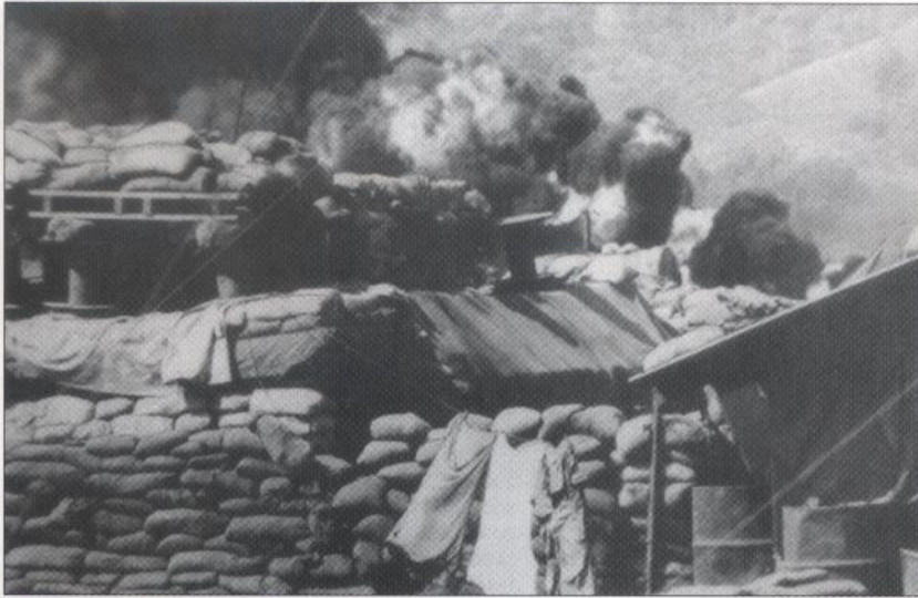
A burning fuel dump set aflame by 122mm rockets. A significant quantity of fuel was stowed on the base for trucks, armored vehicles, weapons carriers, power generators, helicopter emergency refueling, and to burn out latrines – an essential sanitation measure. The bunker in the foreground is built with a stand-off roof above the actual roof with three layers of sandbags stacked atop wooden cargo pallets and set on cable spools for increased protection from artillery, rockets, and heavy mortars.
