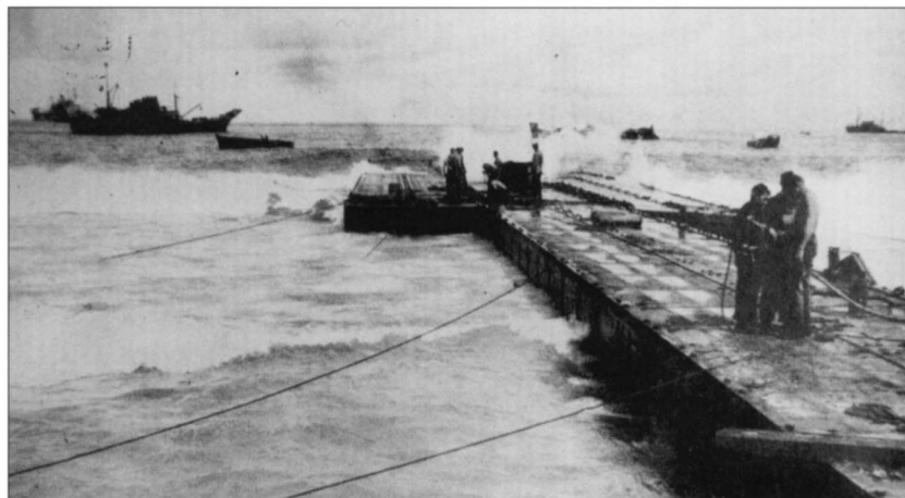
Pontoon causeways were emplaced on both "White 1" and "White 2" reaching to the reef's edge to allow vehicles to roll ashore directly from landing craft without wading and speeding up the landing of equipment and supplies. This "White 2" causeway was damaged by artillery fire on the afternoon of 27 July (J+3). Both causeways were destroyed by a storm on the night of 29/30 July.
