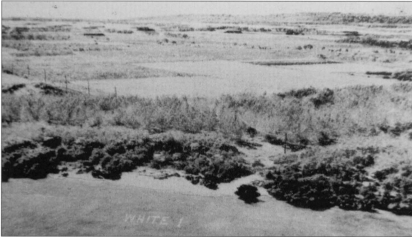
Beach "White 1" on Tinian was 60yds wide with a 200yd-wide approach across the 50yd-wide reef. In this low-tide photograph coral outcroppings and ledges can be seen on the beach. Brush and trees can be seen behind the beach. Note the power line along the road leading to the left. The dark horizontal lines in the distance are aircraft revetments around Airfield No. 1.
