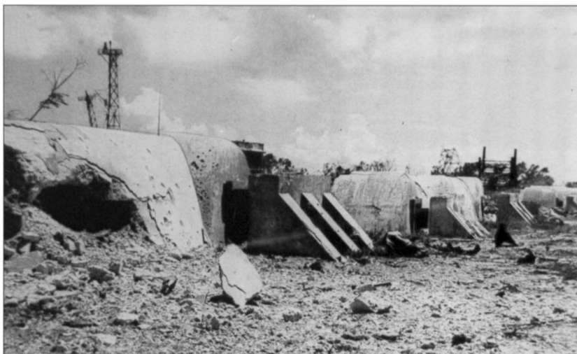
These reinforced concrete air raid shelters were located around Airfield No. 1 on Tinian. They had been destroyed by naval gunfire and dive-bombing. Note the heavily reinforced blast walls protecting the entrances.
