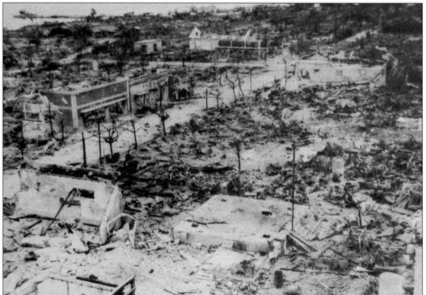
Tinian Town, the island's only community, was virtually leveled to reinforce the Japanese belief that the main landing would occur on the beaches fronting the town. Even most of the concrete buildings were flattened.
