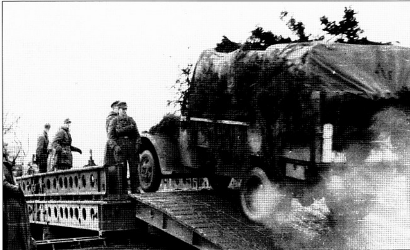
The demolished rail bridge on the Malmedy-Stadkyll rail-line held up the columns following behind Kampfgruppe Peiper's spearhead. It was finally spanned by a J-Gerät bridge, which enabled trucks and other wheeled vehicles to follow. (NARA)
