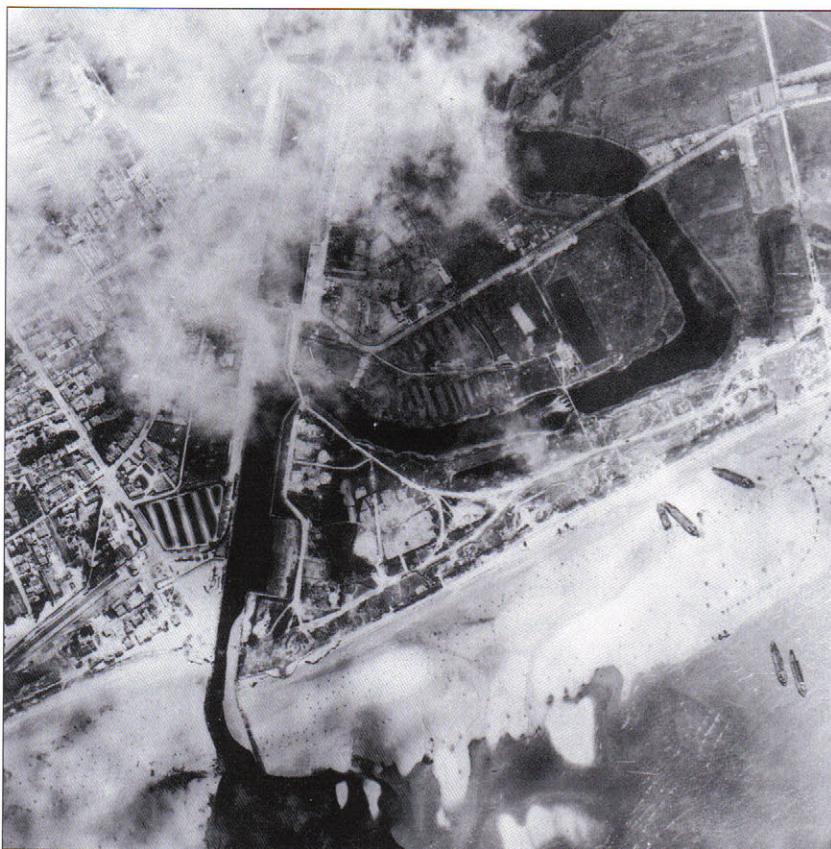
Aerial view of the mouth of the River Seulles at Courseulles harbour, taken just after the assault waves have gone in. On the left of the picture is Nan Green Beach, to the right of the estuary is Mike Red Beach. (Imperial War Museum, CL40)
