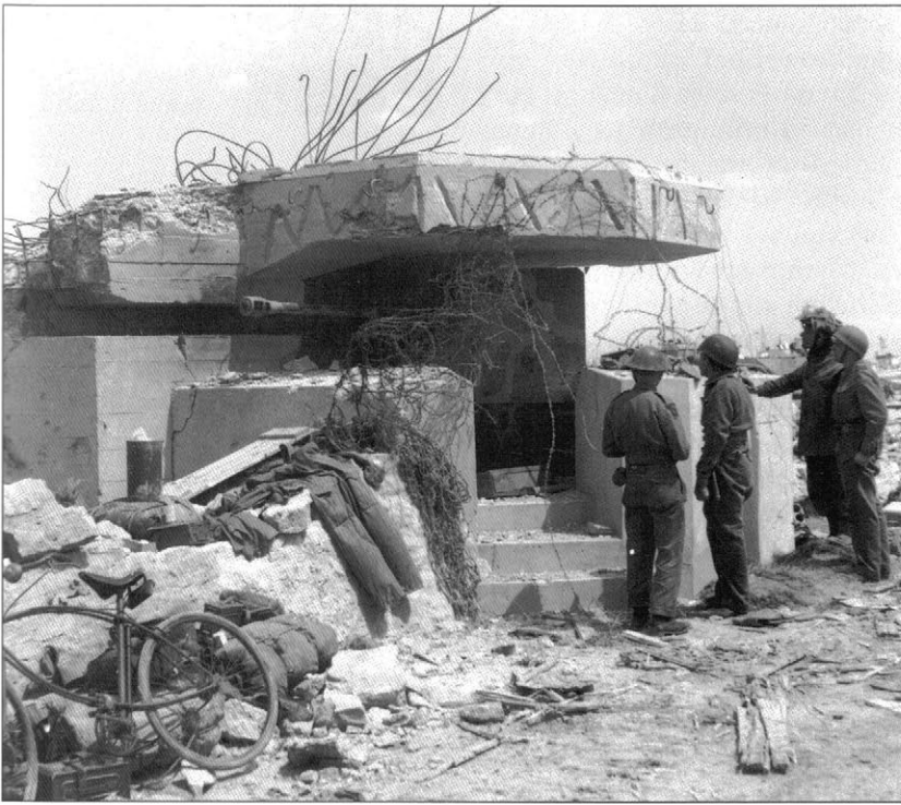
Troops from 50th Division inspect a 50mm gun in its concrete emplacement somewhere along Gold Beach. It has been struck by naval shellfire on its side, but damage seems to have been superficial. It was probably knocked out at close range by assault troops. (Imperial War Museum, B5252)
