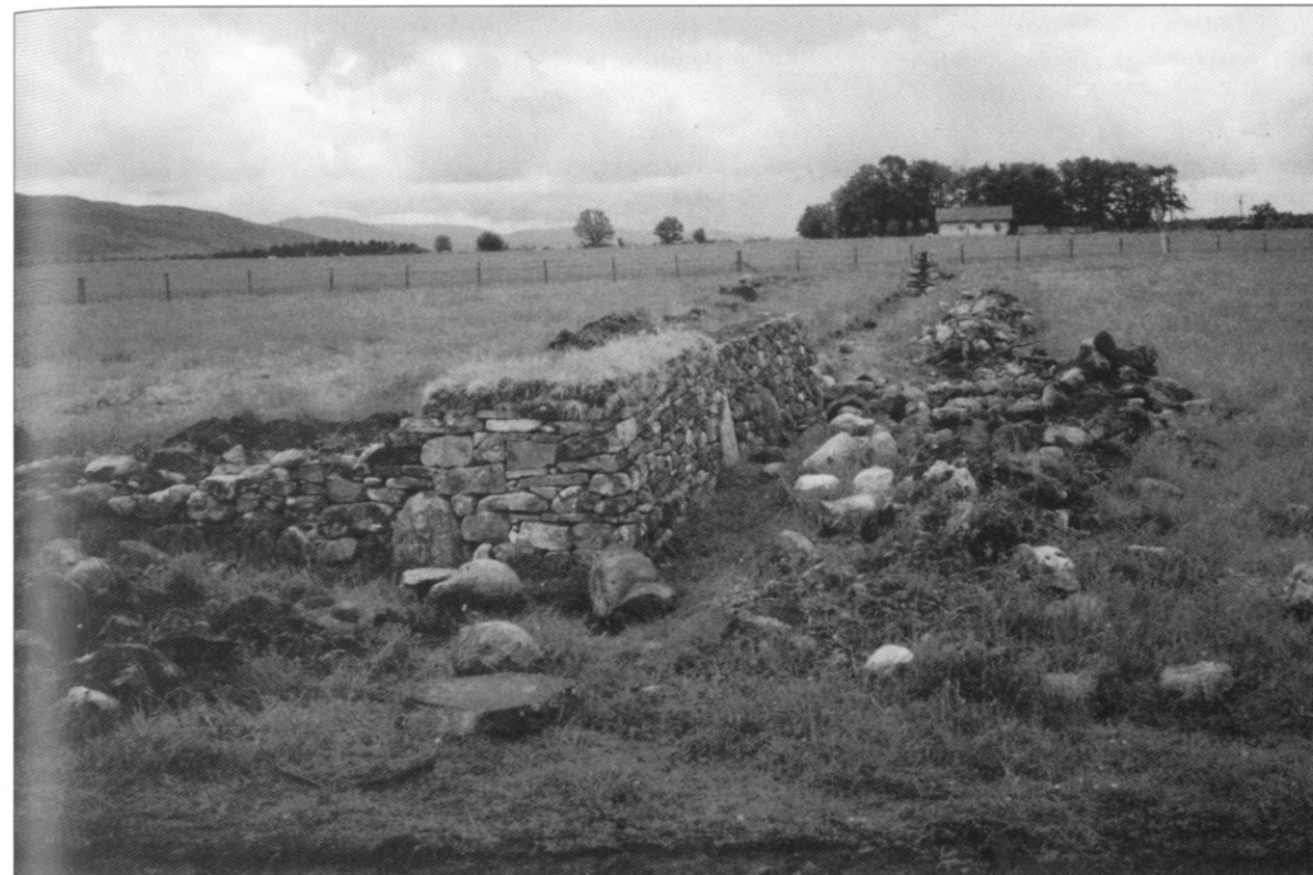
Partially reconstructed Culwhiniac enclosure wall at Culloden. The modern house in the distance marks the far corner of the wall on which the Jacobite right wing was anchored at the outset of the battle.
