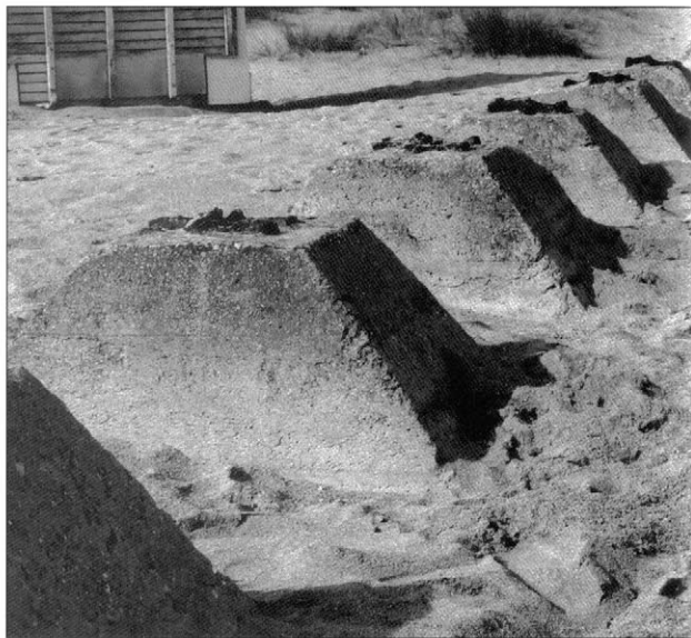
Concrete anti-tank 'dragon's teeth' running alongside the beach huts to the rear of the Casino strongpoint at Riva Bella. The structures are some of the very few remains of the once powerful German beach fortification taken by Capt Phillippe Kieffer and his commandos on D-Day. (Ken Ford)
