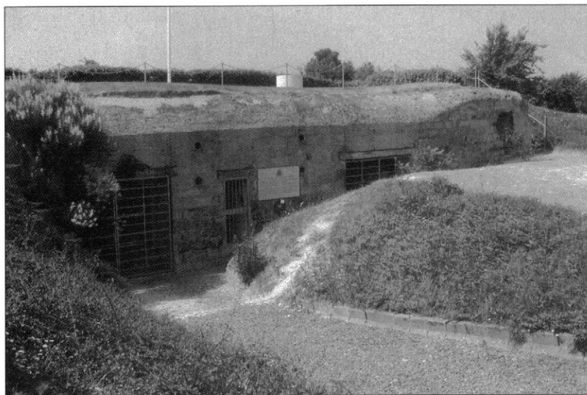
Entrance into the underground complex known to the Germans as Widerstandsnest 17 (Wn 17) and to the British as strongpoint Hillman . The fortified underground position, measuring 400yds by 600yds was located just to the south-east of Colleville, about two miles from Sword Beach. It was captured on D-Day by 1st Suffolks. (Ken Ford)
