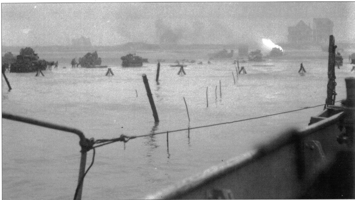
A landing-craft approaches the shore close to the extreme right edge of Queen Red Beach. A Crab flail tank of 22nd Dragoons has been hit and is burning fiercely. Other tanks from 79th Armoured Division are on the beach, as is an armoured bulldozer. A few men are lying in the surf. In the sea can be seen some of the beach obstacles constructed by the enemy. The two prominent villas in the right background still exist, enabling this shot to be located as to the right of strongpoint 'Cod'. (Imperial War Museum, B5111)
