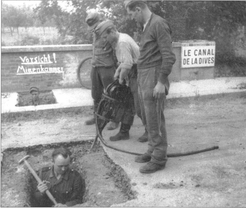
German troops mine a bridge over the Dives Canal before the invasion. The River Dives marked the eastern boundary of the proposed landings of British 6th Airborne Division. (Bundesarchiv, 721/382/32A)
