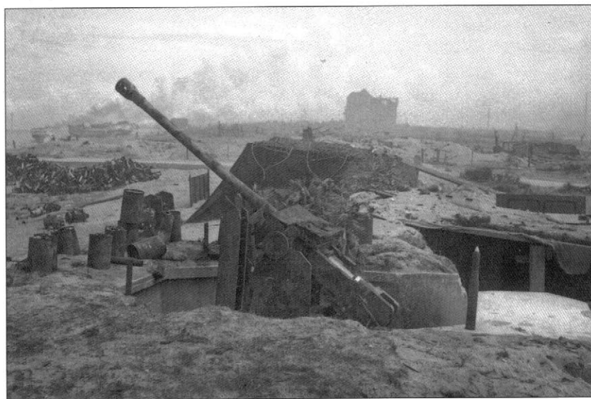
A knocked-out German anti-tank gun pit on the edge of the beach. The gun is a 5cm Kampfwagenkanone in an open emplacement. The wire entanglements and other emplacements in the background give a good indication of the depth of fortifications that existed behind the beaches. (Imperial War Museum, B6379)
