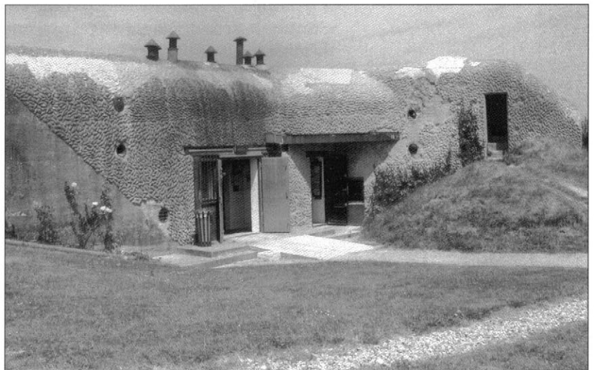
The rear of Merville Battery's Casemate 1, the largest of the four gun positions. To the right is a doorway leading up steps to a 'Tobruk' weapons pit on the roof. Covering the main door is a machine-gun embrasure. (Ken Ford)
