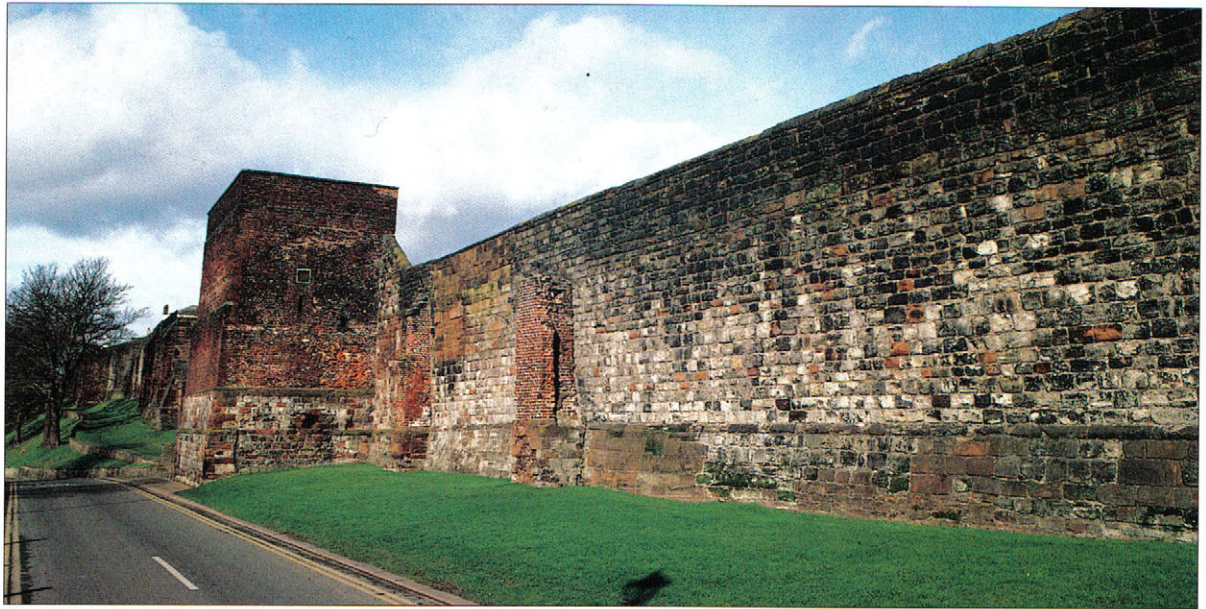
The Tile Tower and part of the City Walls of Carlisle. In 1315 Robert Bruce besieged the town, and despite the use of siege machines the garrison held out, losing only two men. All the Scots achieved was to trample down the cornfields and drive off the livestock.
