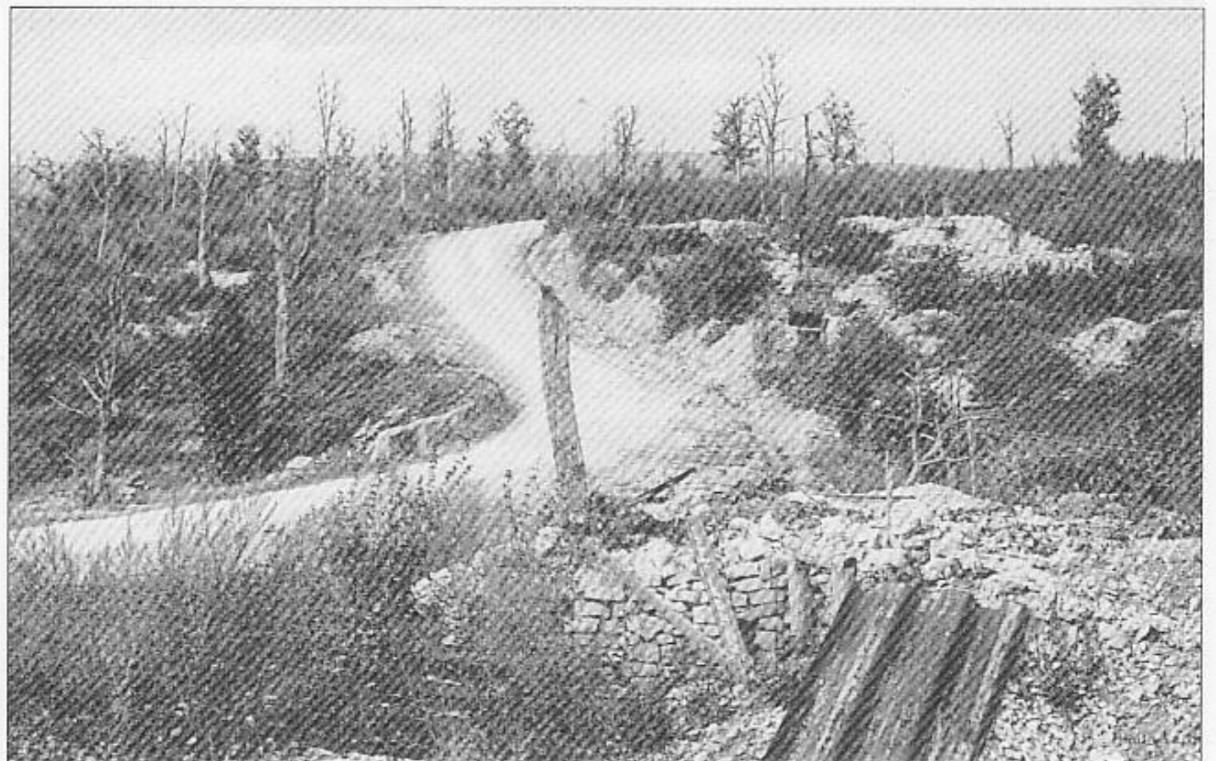
RIGHT The Bois de Tavannes over which many German attacks were launched against Fort Souville. Tavannes fort was bombarded by the heaviest guns: a 420mm round from a 'Big Bertha' penetrating the concrete roof on 7 May.
