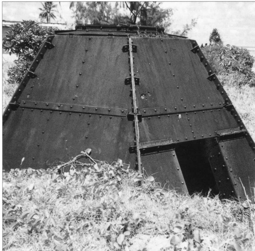
A rusting steel plate command post near Takarongo Point. Originally this two-story structure, constructed of two layers of plate with sand between, would have had a swiveling cupola on top. (Jim Moran)
