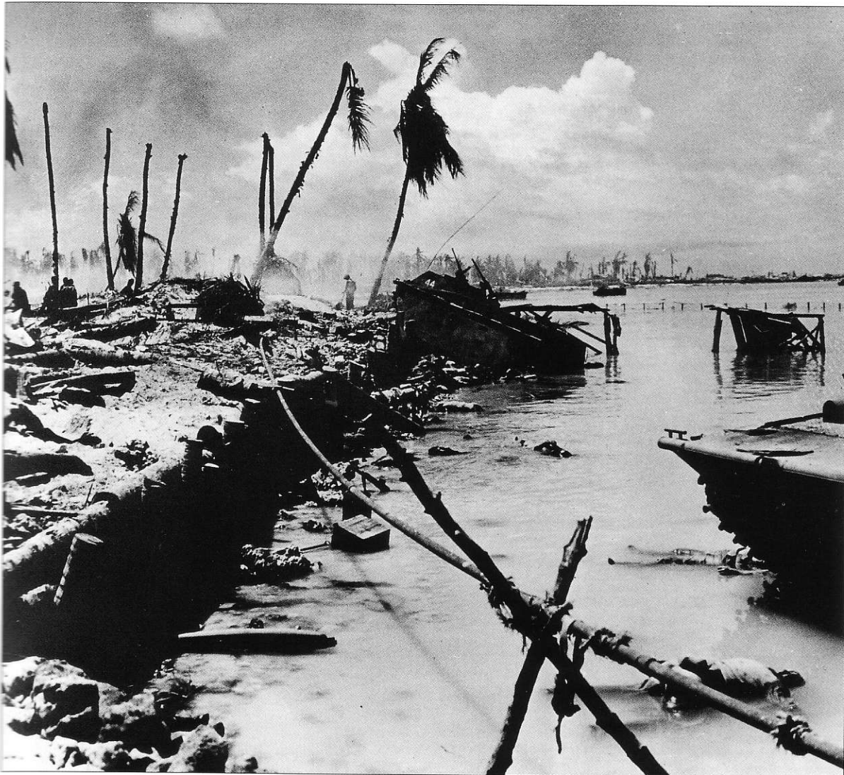
The Japanese caused devastating damage to the amtracs approaching Red Beach 1. Here abandoned LVTs and floating bodies at the log barricade bear witness to the effectiveness of the defenses. (National Archives)
