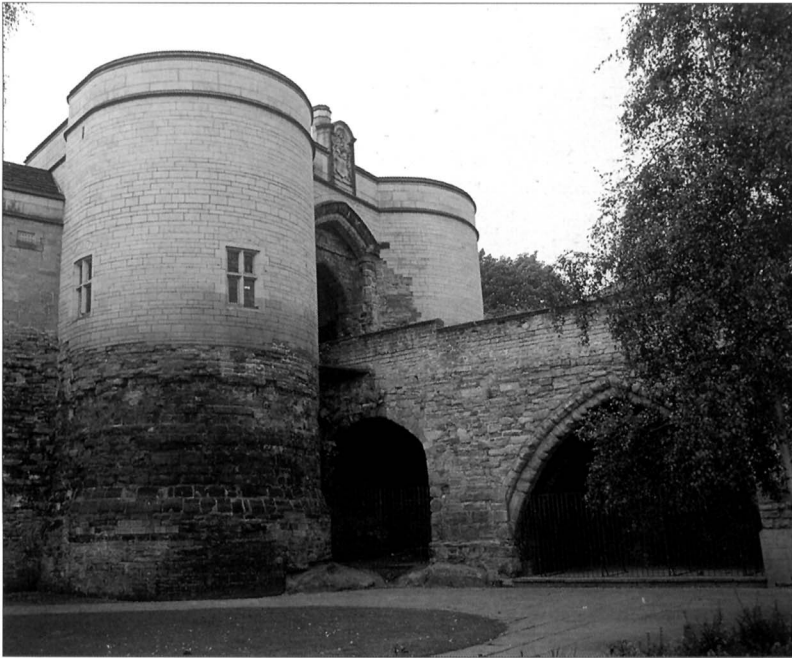
The main gatehouse of Nottingham Castle, heavily restored. Much of the original castle has been destroyed.
