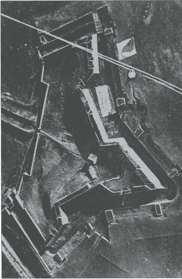
Fort Pardaleras, photographed in 1914. Note how the rear of the fort has no ditch but is connected with the town by a covered way. Today the fort is unrecognisable, having been a prison and an art gallery.
