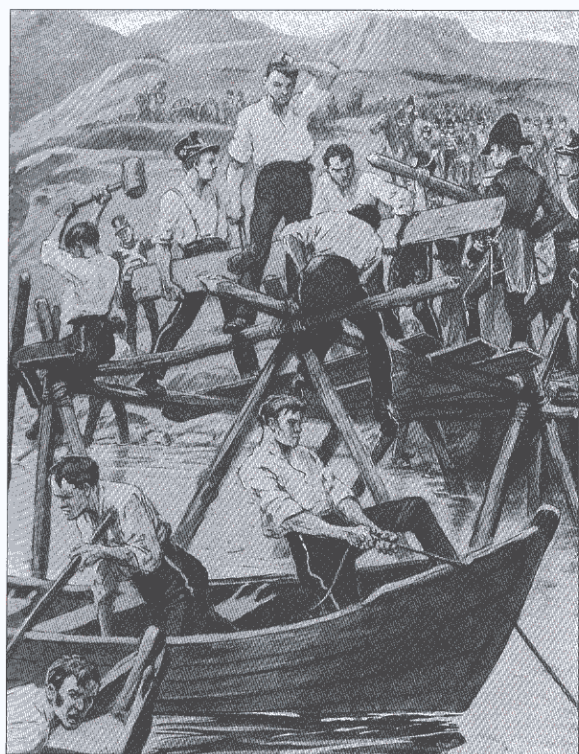
British infantry constructing a bridge over the Guadiana prior to the siege in 1811. The scene would have been repeated in March 1812, when both a pontoon bridge and a 'flying' bridge were constructed over the Guadiana. From a picture by Browne.
