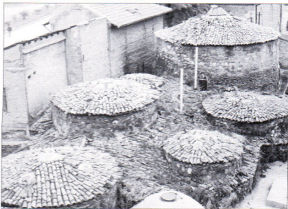
The Orta Hamam or 'Regimental Bathhouse' in Bolu was built during the reign of Bāyazid in the late 14th century. (Author's photograph)
