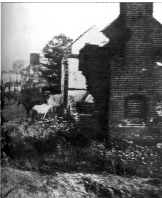
On Willis' Hill, near Marye's Heights, houses came under bombardment. This one brick home was virtually knocked down by the hundredweights of shells which hit it. Others in town suffered a similar fate. When the shelling ceased, Confederates crawled from holes and cellars to resume sniping at Union engineers trying to assemble the pontoon bridges.
