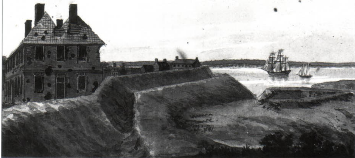
A view of Yorktown, by B Latrobe. This water colour, painted around 1796, shows the still-vacant house of Thomas Nelson (uncle of Governor Nelson and known as Secretary Nelson). In the foreground are the ditch and parapet of defensive works built by the French after the British surrender. At the right is a fleche, an open-backed arrow-shaped work, usually constructed to protect a weak point in the line, or cover a hidden way or ravine. (Courtesy: Virginia State Library, Richmond)
