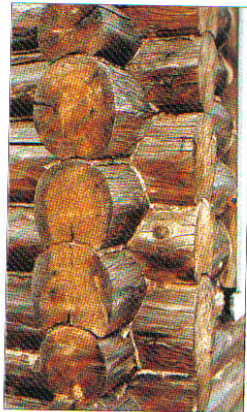
Virtually the same methods of timber construction used in 13th century Russian fortresses are used for some houses in the Russian countryside. This example in Vladimir shows how the tree-trunks were grooved to make a weatherproof fit and to achieve a strong corner. (Author's photograph)
