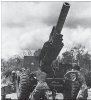
The crew of a 155mm M14A1 howitzer jacks the weapon up on its jack stand, which allowed it to be traversed. If possible, artillery pieces were mounted on level timber platforms to improve their accuracy.
