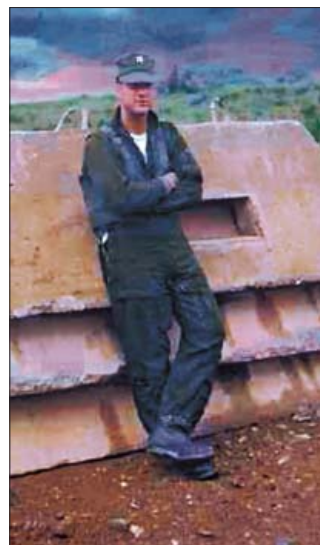
An aviator stands beside prefab contract bunker caps. These were helicoptered into firebases and set over pre-dug, pre-sandbagged bits. (Peter J. Dunne)
