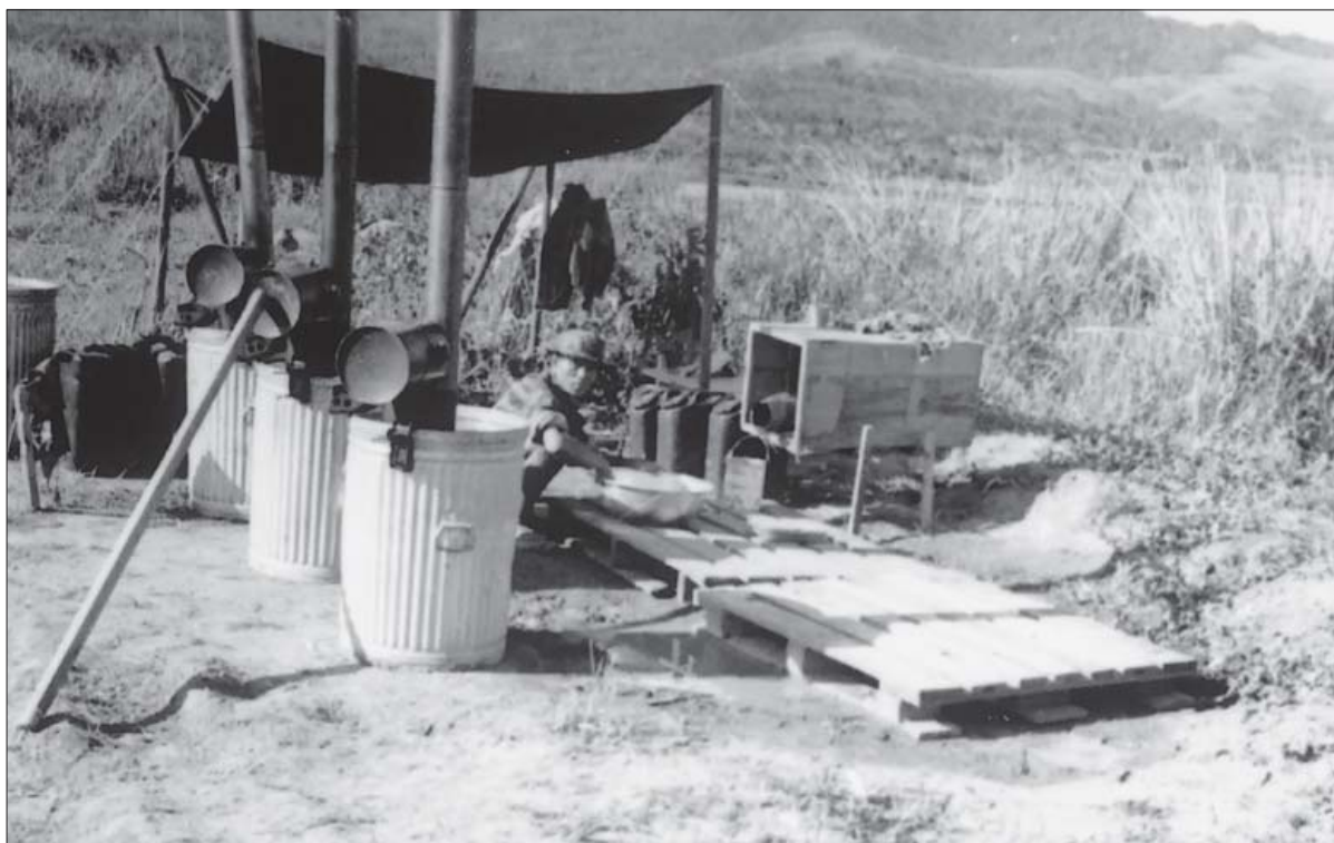
A striker cook cleans a serving bowl at a mess kit washstand made from wooden cargo pallets. The 32-gal. GI cans are fitted with immersion heaters that keep the soap and rinse water cans boiling. (Lee B. Wilson)
