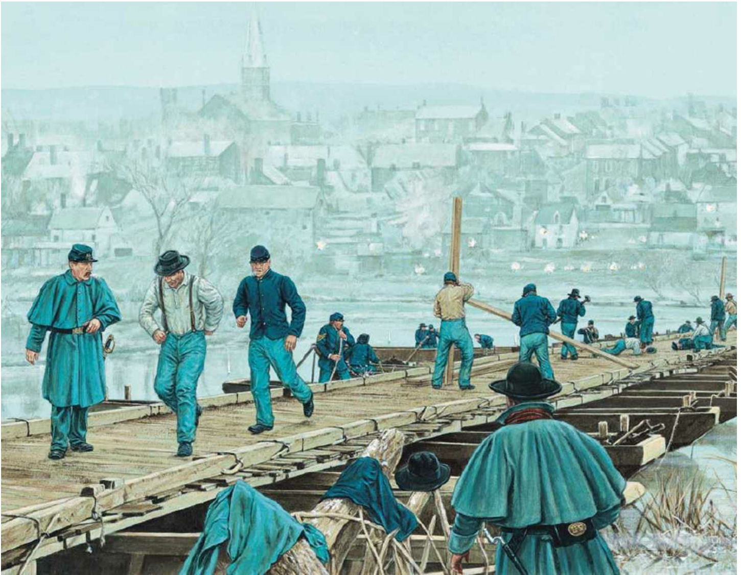
Union engineers laying pontoon bridges across the Rappahannock, by Adam Hook © Osprey Publishing Ltd. Taken from Campaign 63: Fredericksburg 1862.
