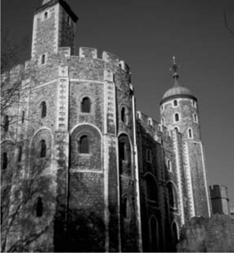
Figure 8. The White Tower, Tower of London, exterior of Chapel of St. John. The white plastered walls of the White Tower were also enriched with pilaster-buttresses joined by arches. The corner turret at the right was slightly enlarged to accommodate a formal staircase, and the large semicircular tower at the left is the outer wall of the apse of the Chapel of St. John. Photograph: Karen Leider.
