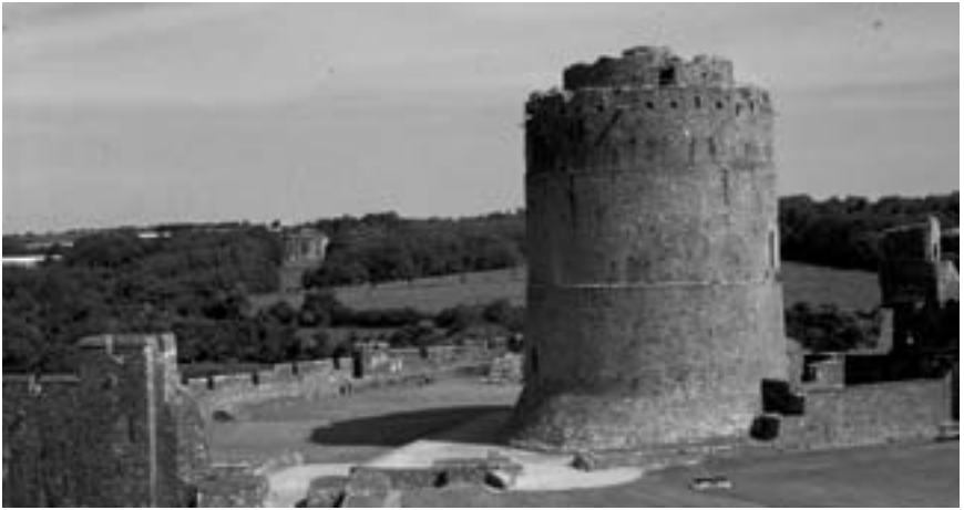
Figure 4. Great tower, Pembroke Castle, Wales. William Marshall built the great tower about 1200 in the most up-to-date style. Round towers entirely of masonry with double fighting galleries had proved to be more effective than the old square towers. The vast open space within the castle walls would have been filled with wood and thatch shelters for people and animals. The foundations and some walls of masonry buildings can also be seen near the great tower. Photograph: Karen Leider.
