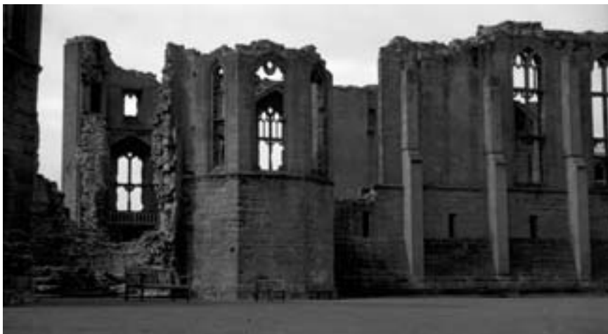
Figure 27. John of Gaunt's Hall, Kenilworth Castle, England. Across the wide courtyard from the great tower (see Figure 10) stands the great hall built in the 1380s. The addition of large windows to the great hall and the private chambers turned Kenilworth into a palace. Photograph: Marilyn Stokstad.
