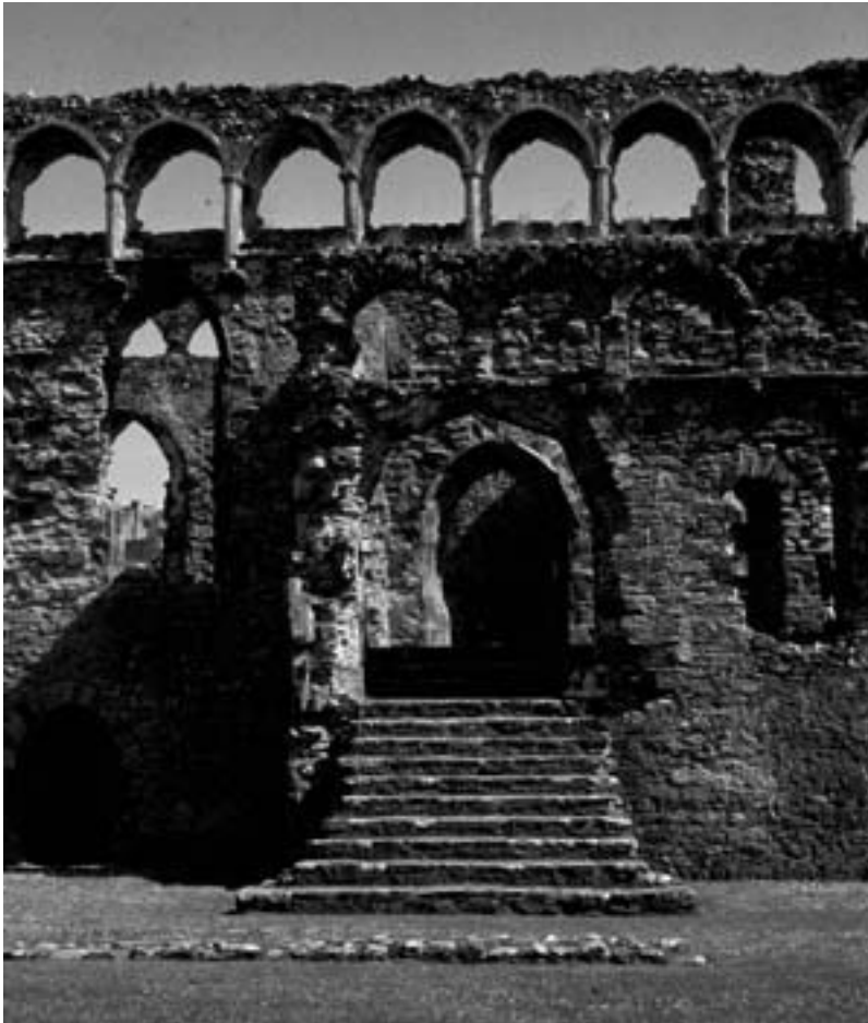
Figure 25. Grand stair, Bishop's Palace, St. David's, Wales. Few of the grand palatial stairways still exist, but the Bishop's Palace boasts of two. The normal medieval stairway was an unimpressive and often difficult tight spiral fit into the wall of the building. Photograph: Karen Leider.
