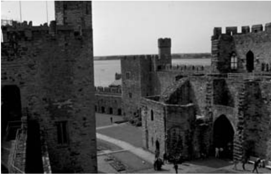
Figure 19. Gatehouse and lower court, Castle of Caernarfon, Wales. Built at the end of the thirteenth century, Caernarfon was the English king's governmental center in northern Wales. At the far right of the photograph is the King's Gate, the most complex gate built in medieval England and Wales. The lower courtyard contained the residence of the governor, a residence for the queen, and the great hall and the kitchens. The castle was accessible from the water and two watergates opened into this lower court. Photograph: Karen Leider.
