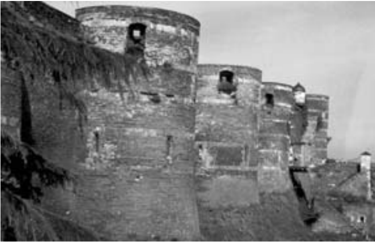
Figure 17. The Castle of Angers, France. Even when lowered to form bastions for cannon, the towers of the Castle of Angers amaze us with their huge size. The banded appearance of the masonry represents an efficient building technique using bonding and leveling courses of different materials. Developed by Roman and then Byzantine engineers, the technique was adopted by Muslims and Christians and often used for its decorative effect. Photograph: Marilyn Stokstad.
