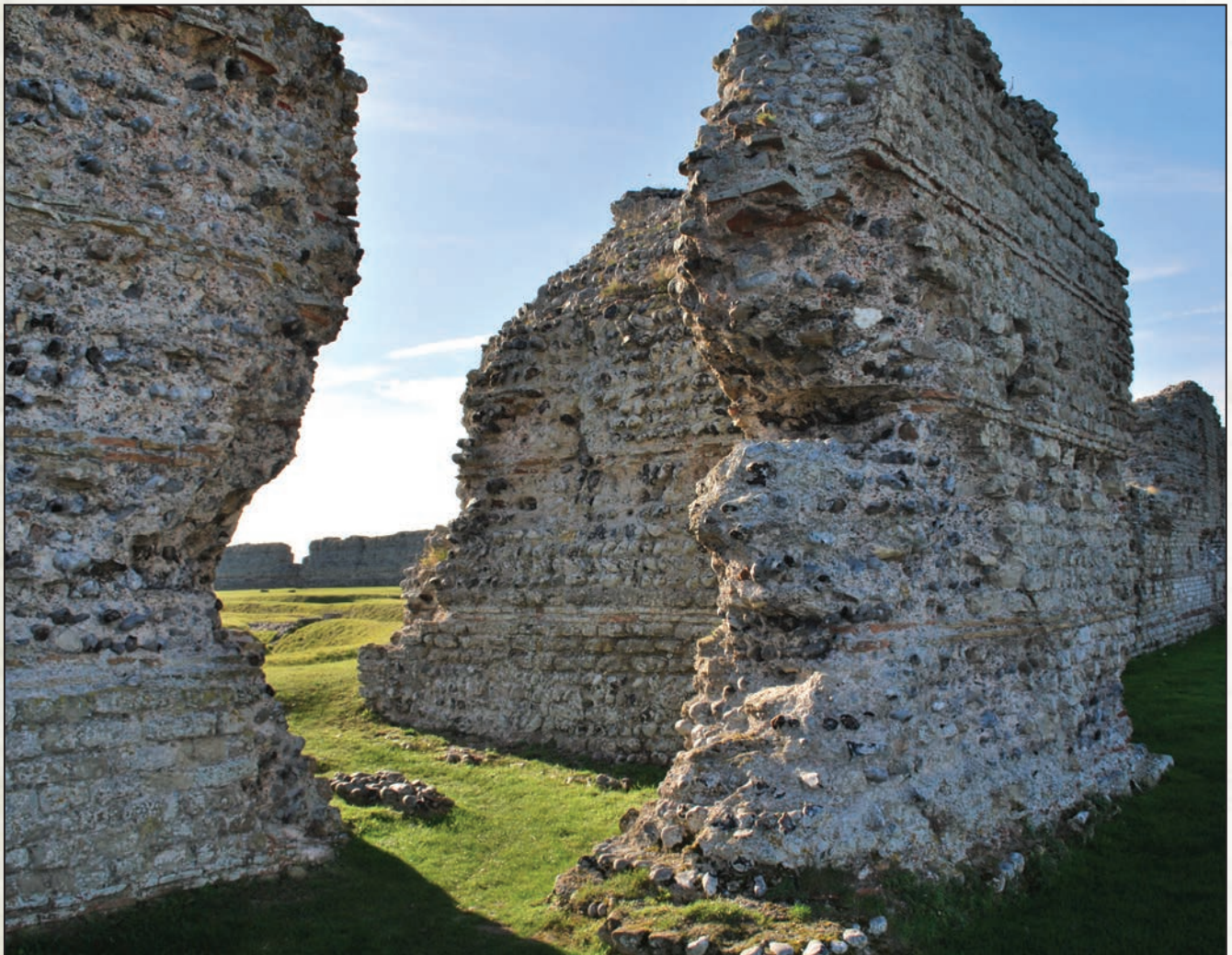
How the Roman beachhead site looks today. The Romans built a town, amphitheatre and triumphal arch there. The arch was eventually pulled down and a Saxon Shore fort put up to keep the English out. These walls are the remains of the fort.
