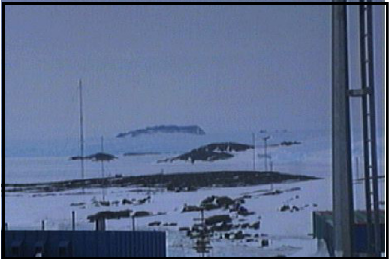
Hatsumi Base Early Construction
