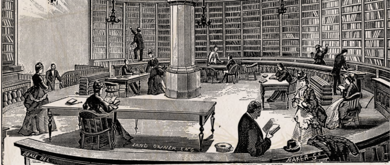
THE BOOK ROOM IN THE OLD WATER TANK.
